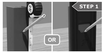
Marking the rail bracket placements on posts can be done either with a tape measure OR our bracket template.
