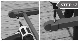
Fasten the bracket cups to the rails at both ends with #14 Tek screws.
