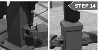
Attach the four rail cups to the four backer plates with #14 Tek screws. Use a rubber mallet to tap the post caps into place to finish the section.
