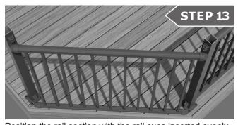
Position the rail section with the rail cups inserted evenly into all four backer plates.
