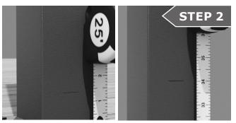
Measure 1-3/8" from the top of the fange and make a pencil mark at that height. Then place a pencil mark at 34" from the top of flange.
