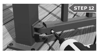
Attach the bottom rail to the bracket cup with a #14 Tek screw.
