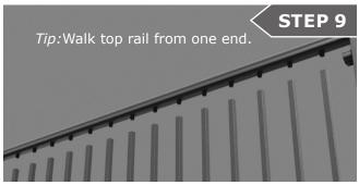
Drop the top rail onto the balusters and top brackets, adjusting the balusters as needed to insert each rail nub.
