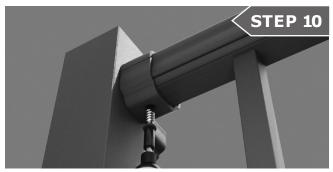
Drive a #14 Tek screw into the underside of each top rail bracket.
