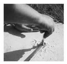
Install the connector nut on top of the stainless steel anchor and tighten. Use the 13/16" wrench.
