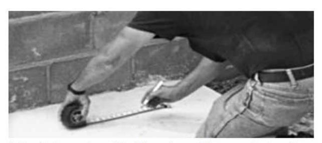
1. Locate the center points of the columns. Make sure the layout and slab are square. NOTE: The concrete slab needs to be a minimum of 5" thick. The concrete footing must be a minimum of 2'x2'x2' and needs to reflect the local building code requirements. Concrete must be a minimum of 2,000 psi.
