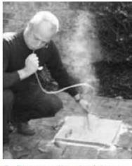
Remove the dust from the hole to ensure a clear insertion of the stainless steel anchor.
