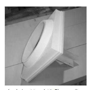
11-12. Locate the column cap shown in photos 11 and 12. Place on the column and feed the threaded rod through the hole in the center of the plate with the welded angle.
