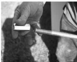
**8.** Attach a connector nut to the threaded rods and then attach the 6" inch stainless steel threaded section to the top of the connector nut.
