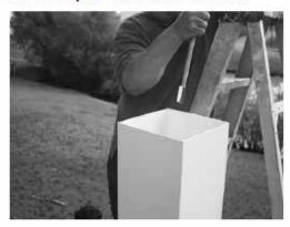
Lower the threaded rod into the column and engage the coupling nut on the bottom.
