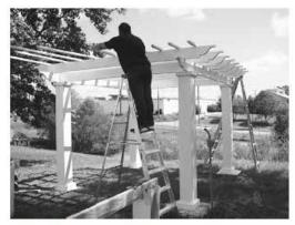
**19.** Set the clutch on the drill to ensure that the screw head does not dimple the top surface of the purlin. Continue across the top of the rafters until all purlins have been installed.
