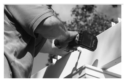
**15.** Install the rafter supports with the decorative rafter tails on the opposite side of the aluminum angle using 2.5" hex head stainless steel self-tapping screws. Set clutch on the drill so the screw is not stripped.
