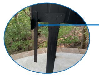
Position the stair strap and fasten to the deck using the Evolution 3/4" Self-Drilling Screws
