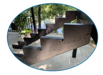
Stringers full assembled and anchored to the deck with the Evolution Stair Strap and anchored to the concrete with the Evolution Anchor Bracket.
