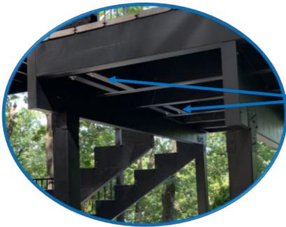
If anchoring to a landing, install blocking and attach the anchor bracket thru the blocking using 3/8" bolts, nuts, and washers.
