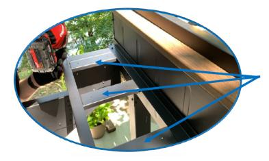
The blocking every 10" On-Center can be used for railing post attach-ment and stair tread attachment.
