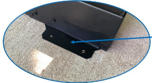
Attached the anchor bracket to the bottom of the stringer using the Evolution 3/4" Self-Drilling Screws.
